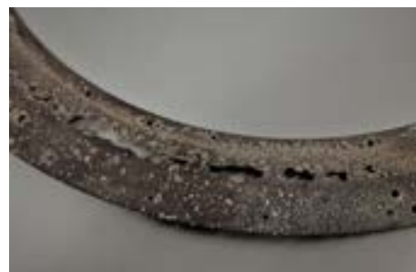
Figure 2. (b) and (c) Part of the turret mounting assembly, heavily corroded showing through-thickness corrosion holes.
